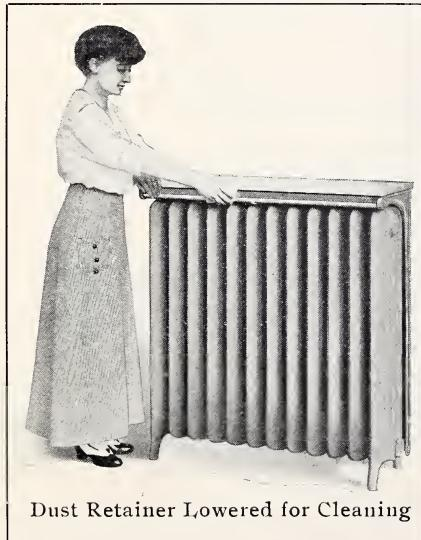
Dust Retainer Lowered for Cleaning
